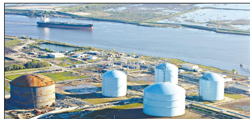
El Paso's LNG import terminal at Elba Island: the US natural gas producer and distributor is planning to split out its upstream, exploration and production entity.
